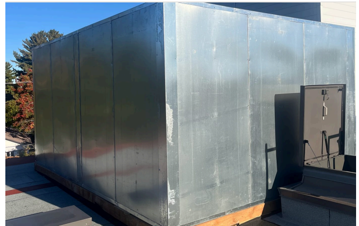
Sound barrier installed around rooftop mechanical equipment.
