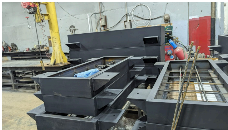
Steel frames in the shop and bases installed on their isolators.
